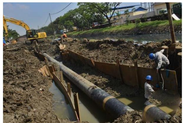
**Gambar 3.** Pemasangan pipa di bawah tanah (under ground)
