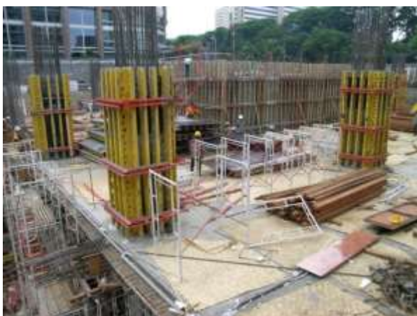
Gambar 2 Bekisting semi sistem Sumber: www.strong-indonesia.com
