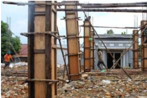
Gambar 1 Bekisting konvensional Sumber: www.ilmunyaorangipil.blogspot.com
